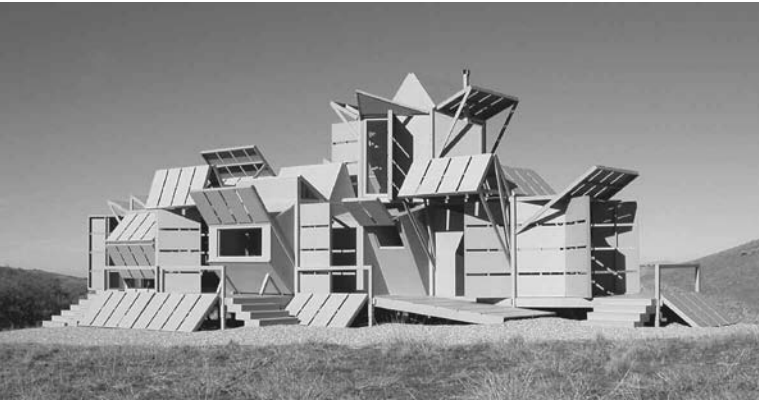
Automatically Adjustable Sunshades: The “M-House,” Gorman, California. Designed by Michael Jantzen. (Photo supplied by Michael Jantzen.)
